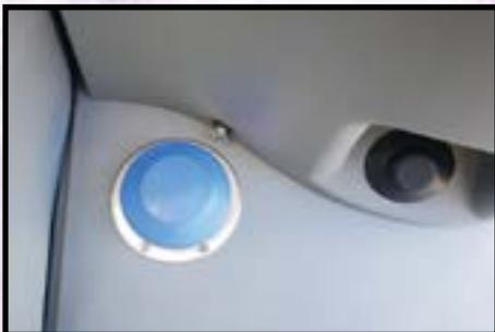
Foot pump provides flushing operation for toilet.
